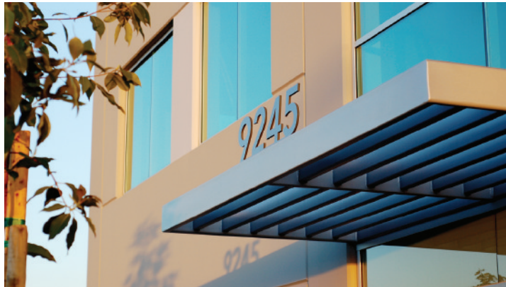
Local presence: HQ in University Research Park, data-center space in airport area
